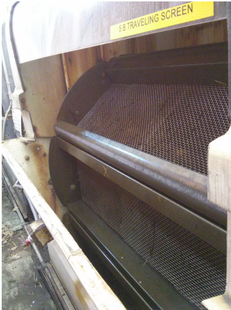
Figure 9-1: Schiller Station's Unit 5 Intake Screen
