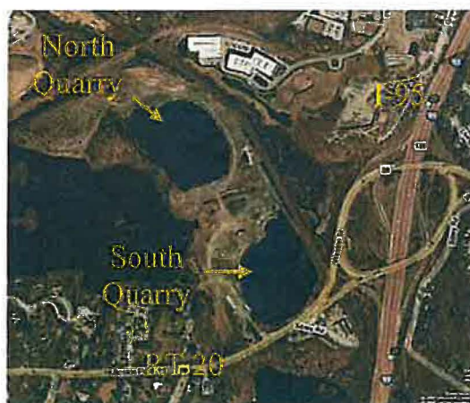
Site Aerial Photo
