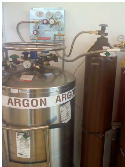
Figure 2. The argon manifold and backup tanks
