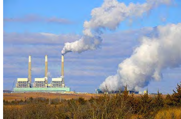
Figure 1: Westar's Jeffrey Energy Center coal-fired generating facility.
