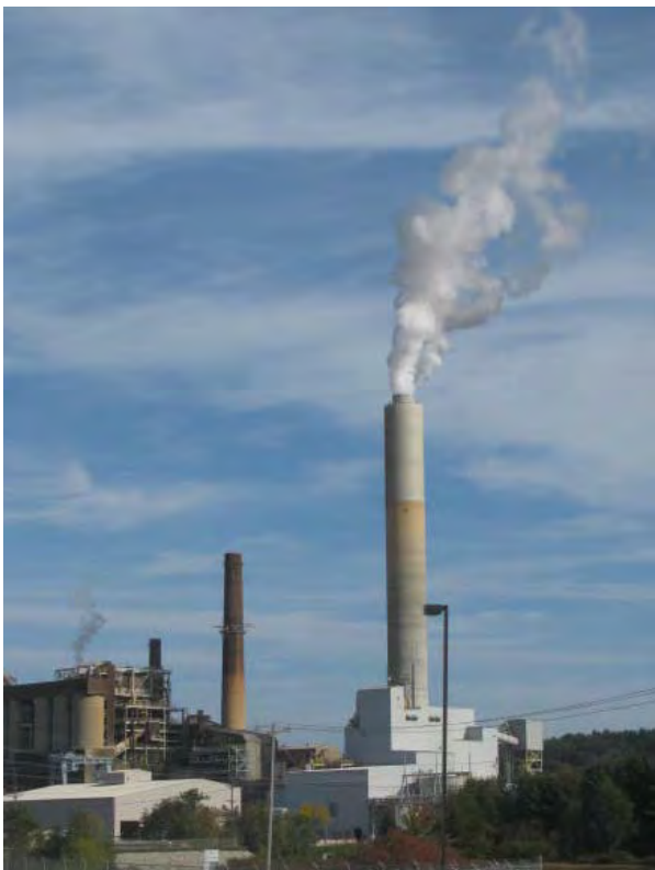
Scrubber in Operation
