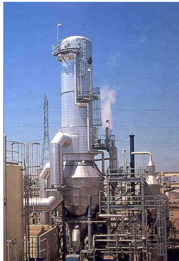
Figure 2. Brine Concentrator. Courtesy Veolia/HPD
