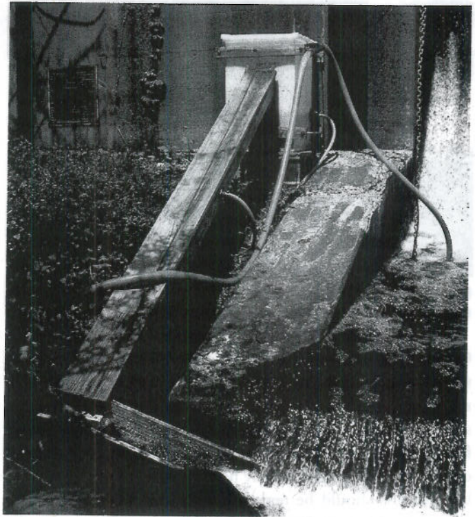
Elver ladder on a small river in western Massachusetts. The hose provides an attractant flow, eels crawl up the ramp into a holding tank, and the tank is emptied on the upstream side of the dam. Ethan Nedeau
