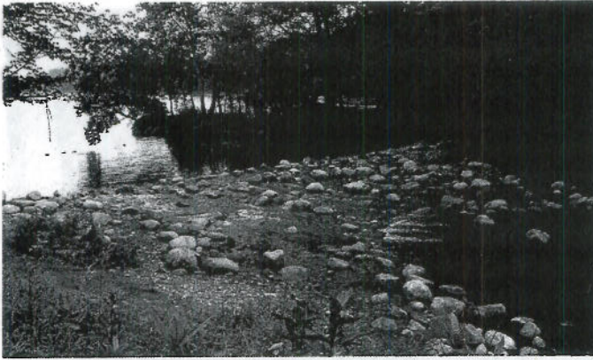
Rock ramp at the outlet of Sennebec Pond in Union, Maine, which replaced a dam but still maintains pond levels. Eric Hutchins
