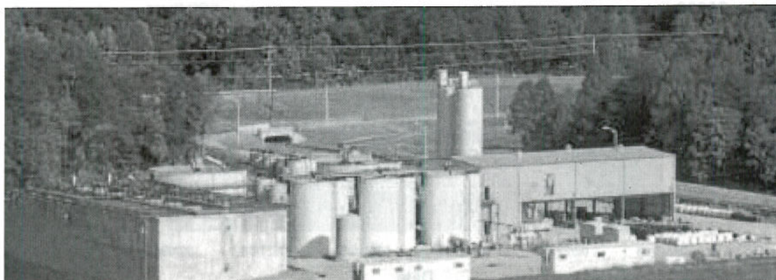
Figure 6: Belews Creek WWTS
