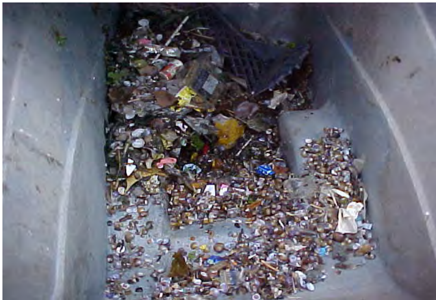
Figure 6-2 Man-made debris collected from a cooling water intake
