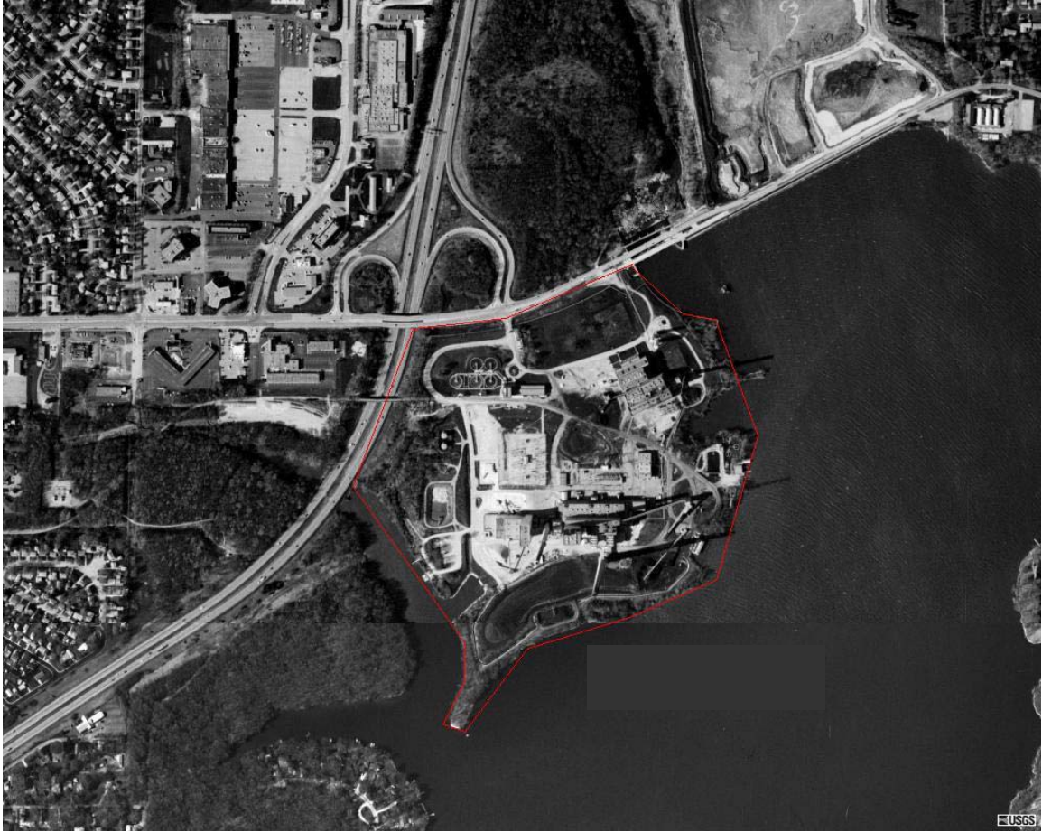
Figure 5-7 Space constrained site; Plant No. F390
