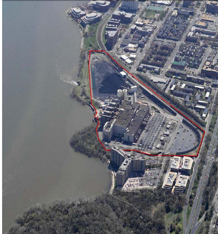
Figure 5-5 Space constrained site; Plant No. F235
