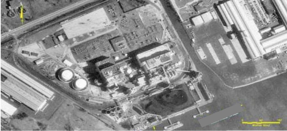
Figure 5-1 Space constrained site; Plant No. F465
