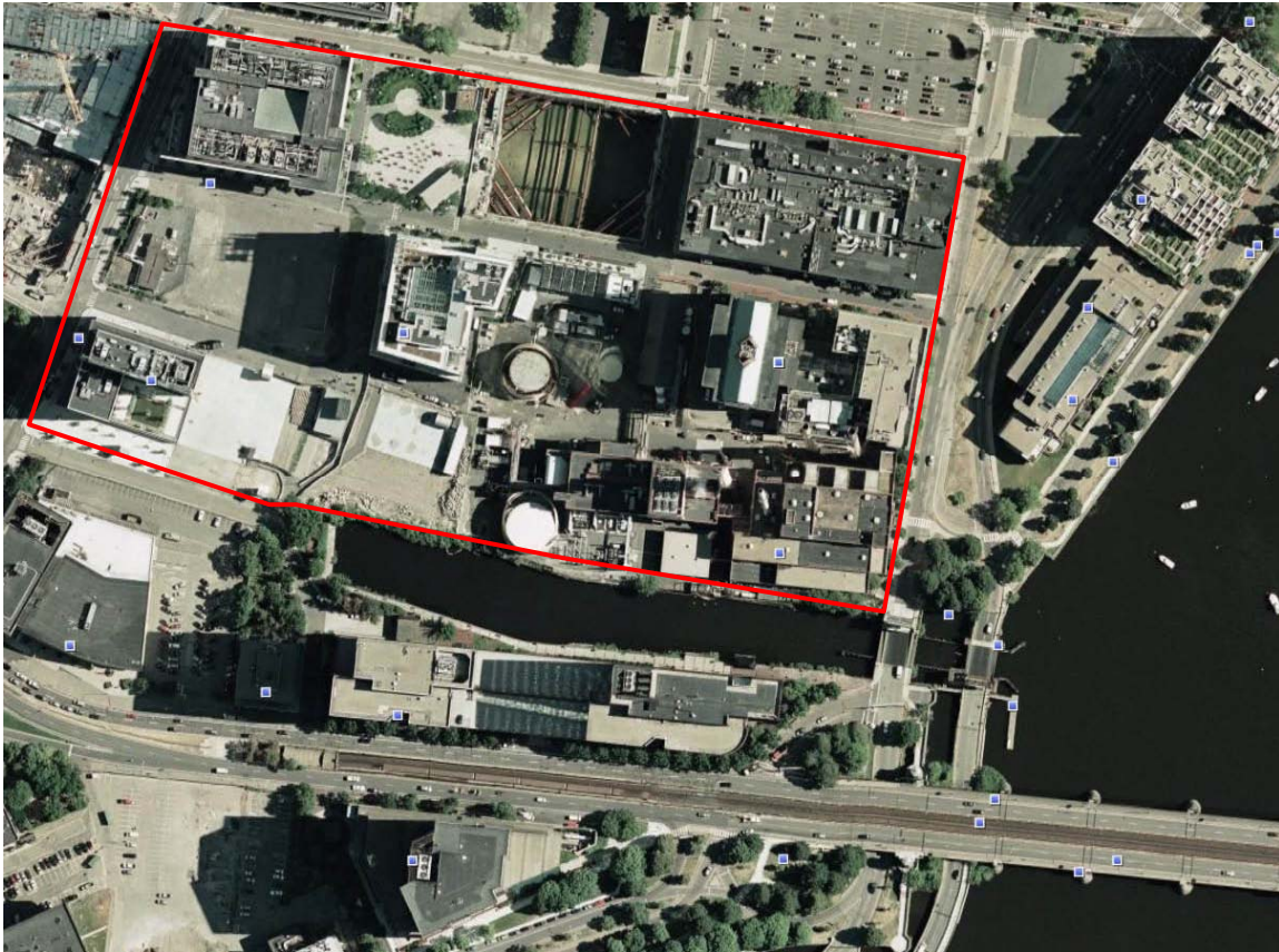
Figure 5-4 Space constrained site; Plant No. F124
