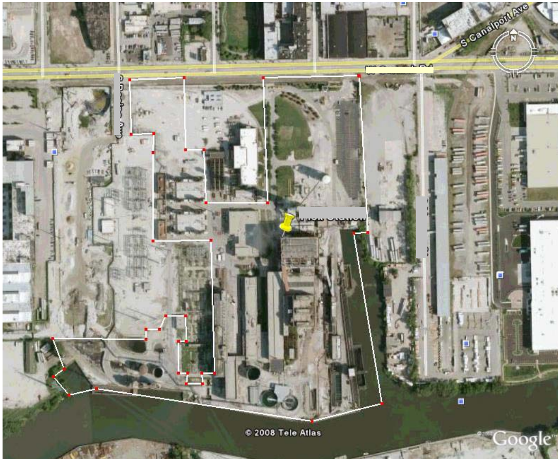
Figure 5-3 Space constrained site; Plant No. F382
