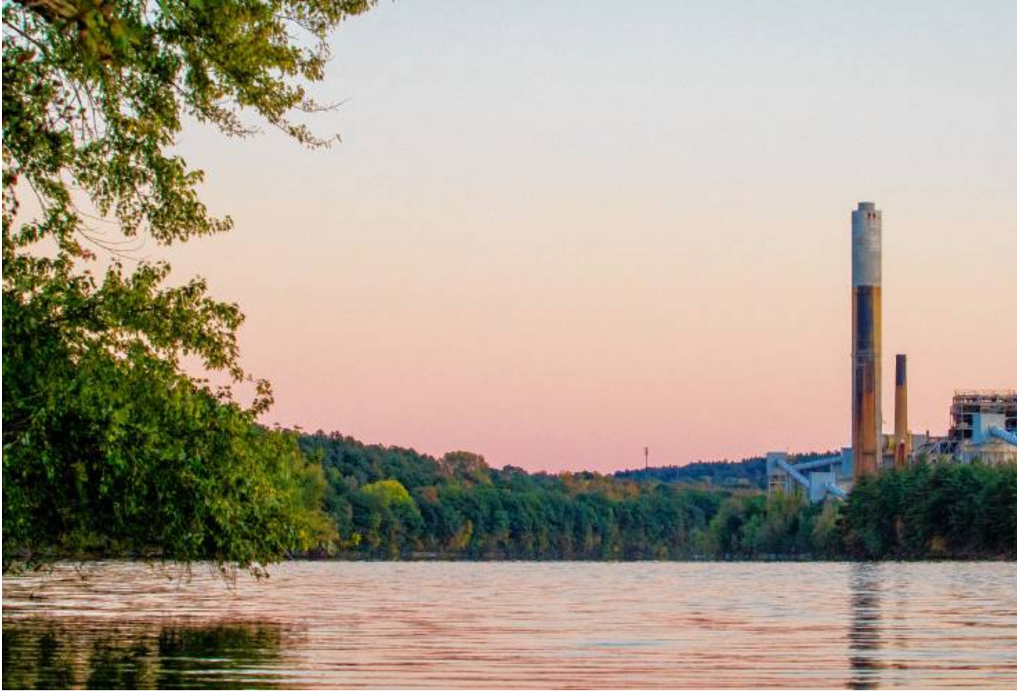
The Merrimack Station power plant in Bow is seen at dusk on Thursday, Oct. 12, 2017. (ELIZABETH FRANTZ / Monitor staff)
