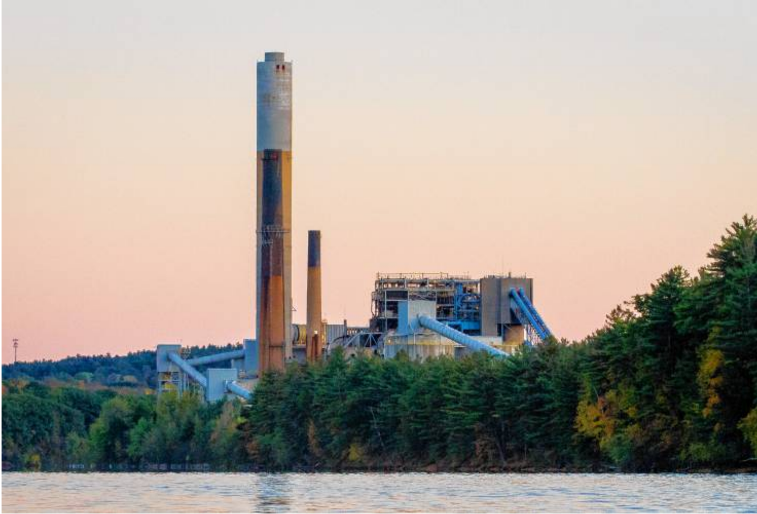
The Merrimack Station power plant in Bow is seen at dusk on Thursday, Oct. 12, 2017. (ELIZABETH FRANTZ / Monitor staff)
