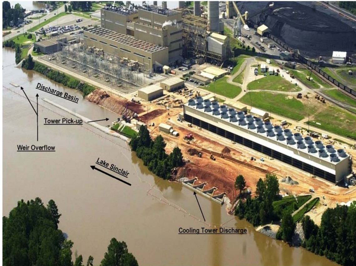
Figure 21-2 Configuration/Design of Plant Branch Cooling Tower System
