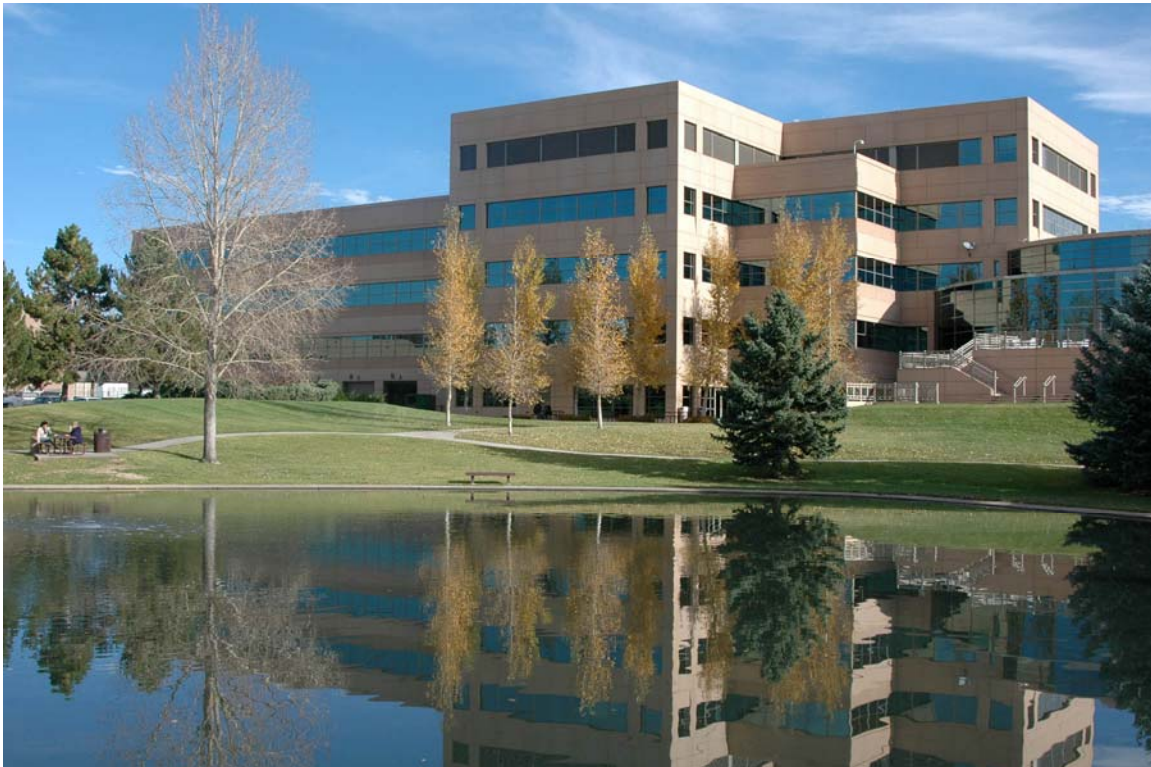
Figure 1-1 Tri-State Transmission and Generation Association Headquarters in Westminster, Colorado
