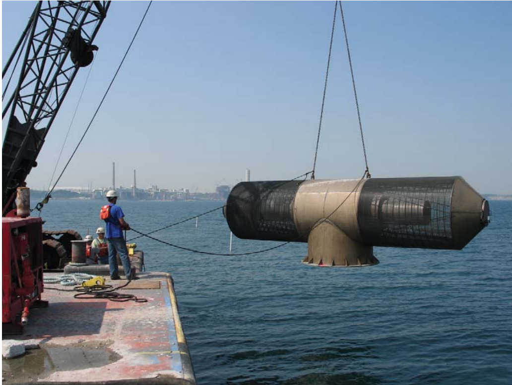
Figure 23-5 Wedge-Wire Screen Installation at Off-Shore Intake Location
