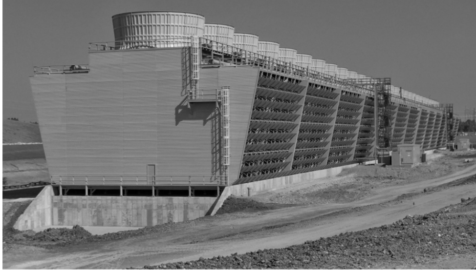
Figure 15-8 BFN new Cooling Tower 7 (under construction)
