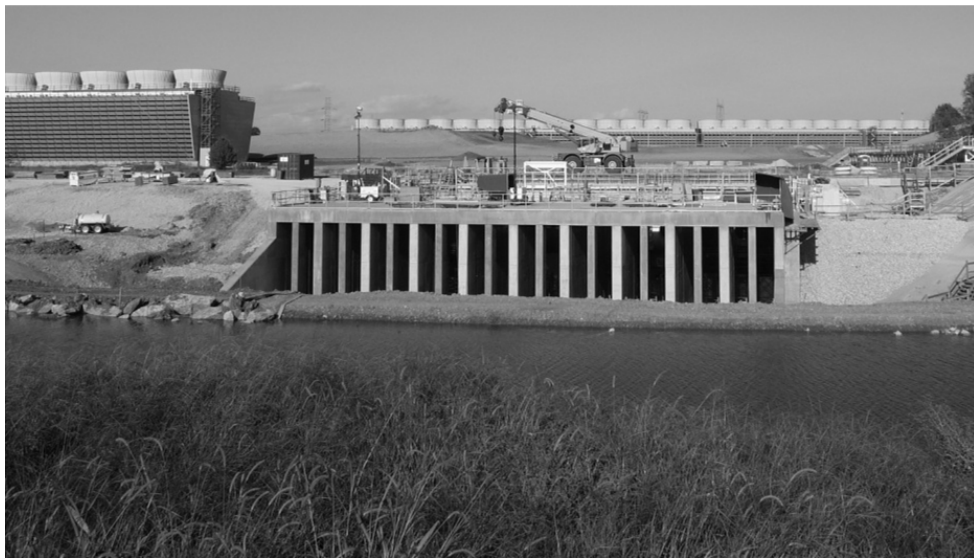
Figure 15-9 BFN new pumping station for Cooling Tower 7 (under construction)
