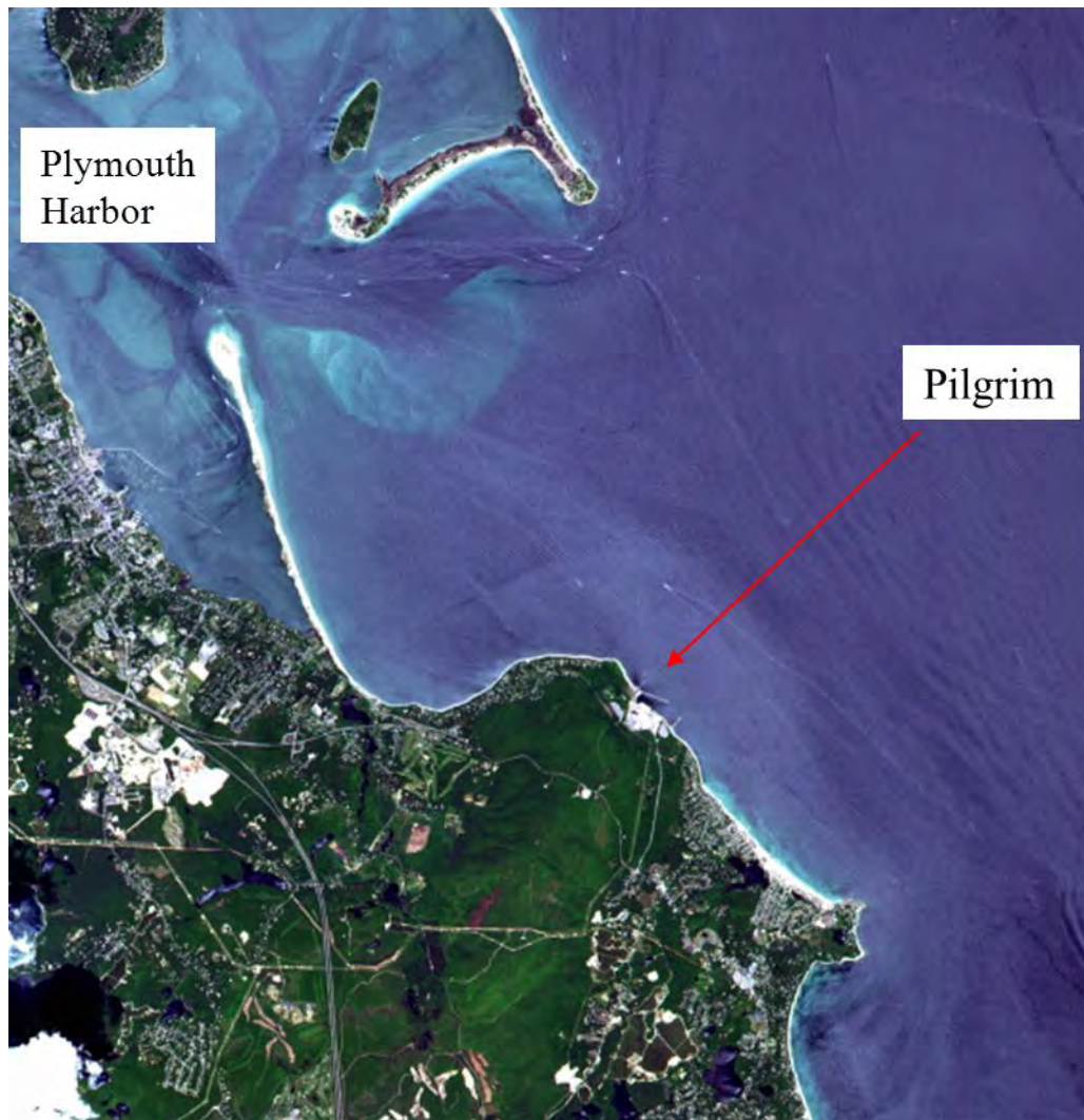
Figure 22-15 Pilgrim Power Plant, just south of Plymouth, Massachusetts
