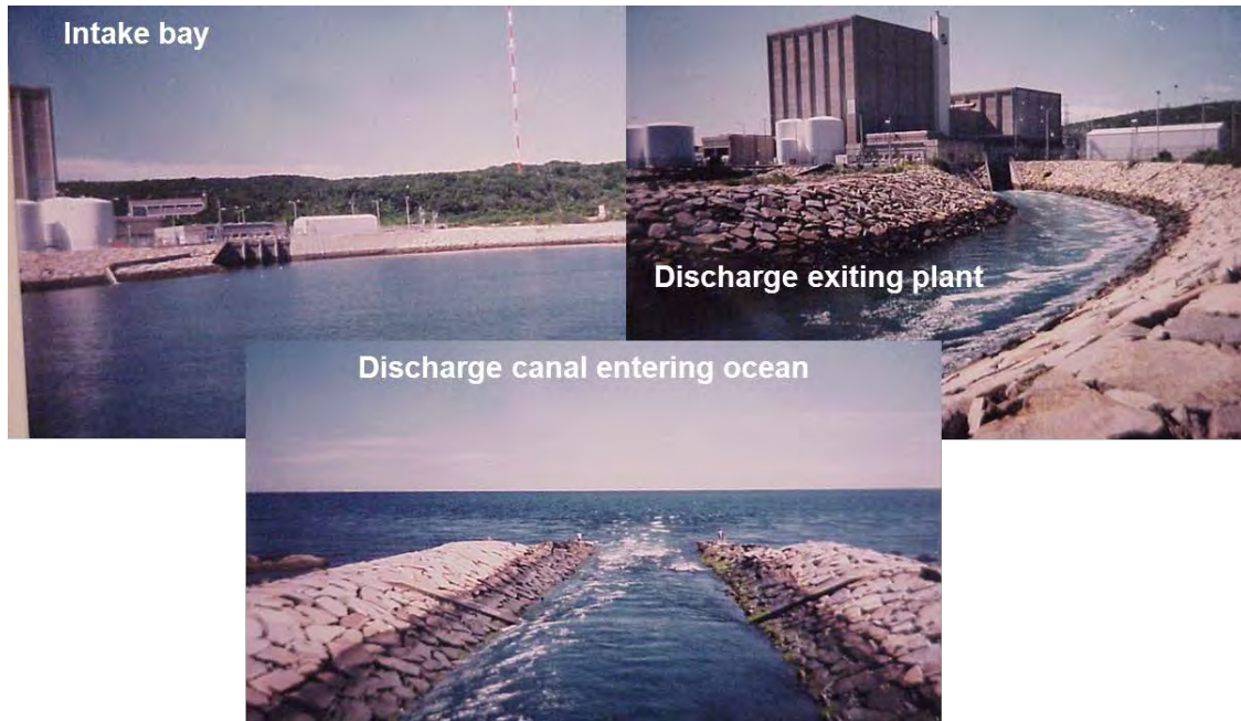
Figure 22-16 Photographs of Pilgrim Power Plant cooling water intake bay and discharge canal into Massachusetts Bay
