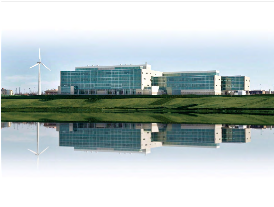
Figure 1-1 Great River Energy’s facility in Maple Grove, Minnesota
