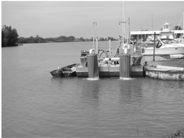
Figure 4-2 Test Facility in Place in the Portage River (facing west)
