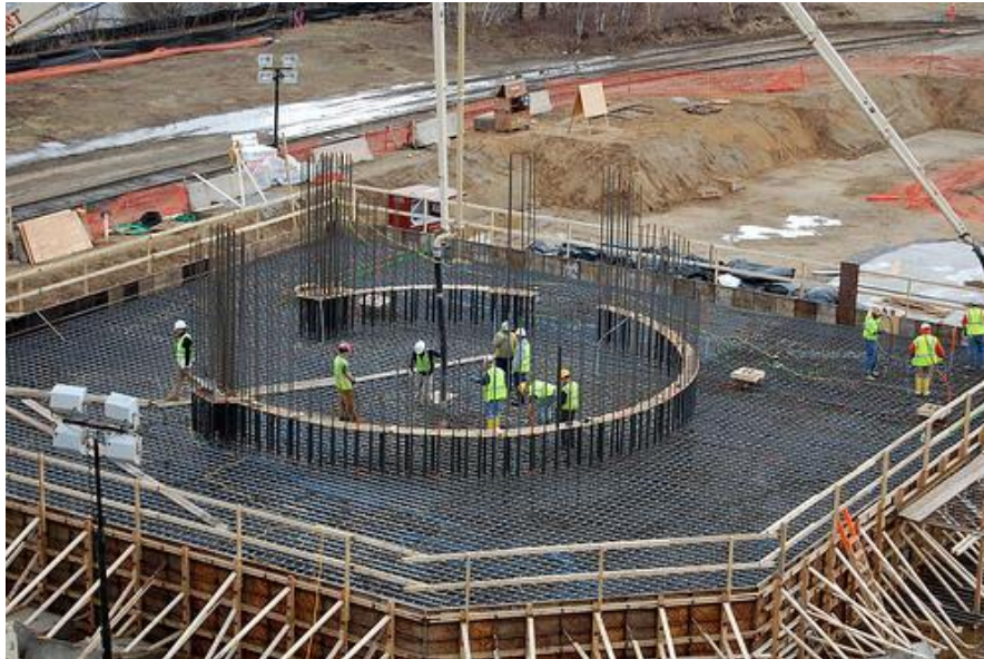
Figure 1: Construction of the Chimney Foundation, Part of the Scrubber System 3
