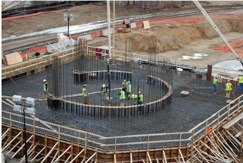
Figure 9: Construction of the Scrubber System Chimney Foundation 4
