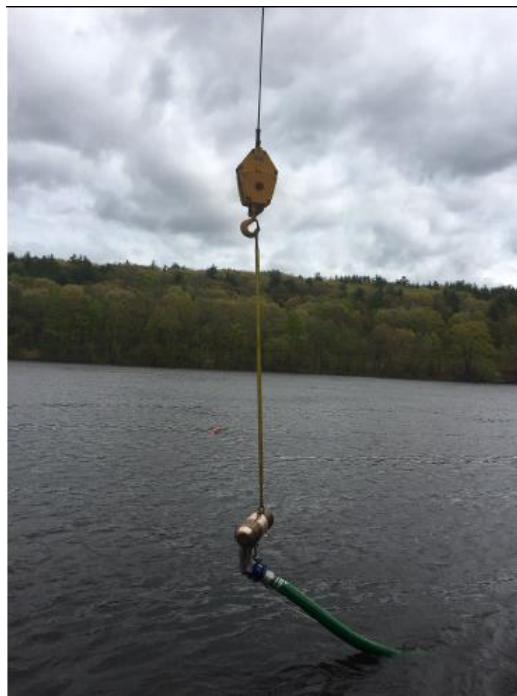
Figure 5 – Photo of Pilot Test Screen Installation in Merrimack River
