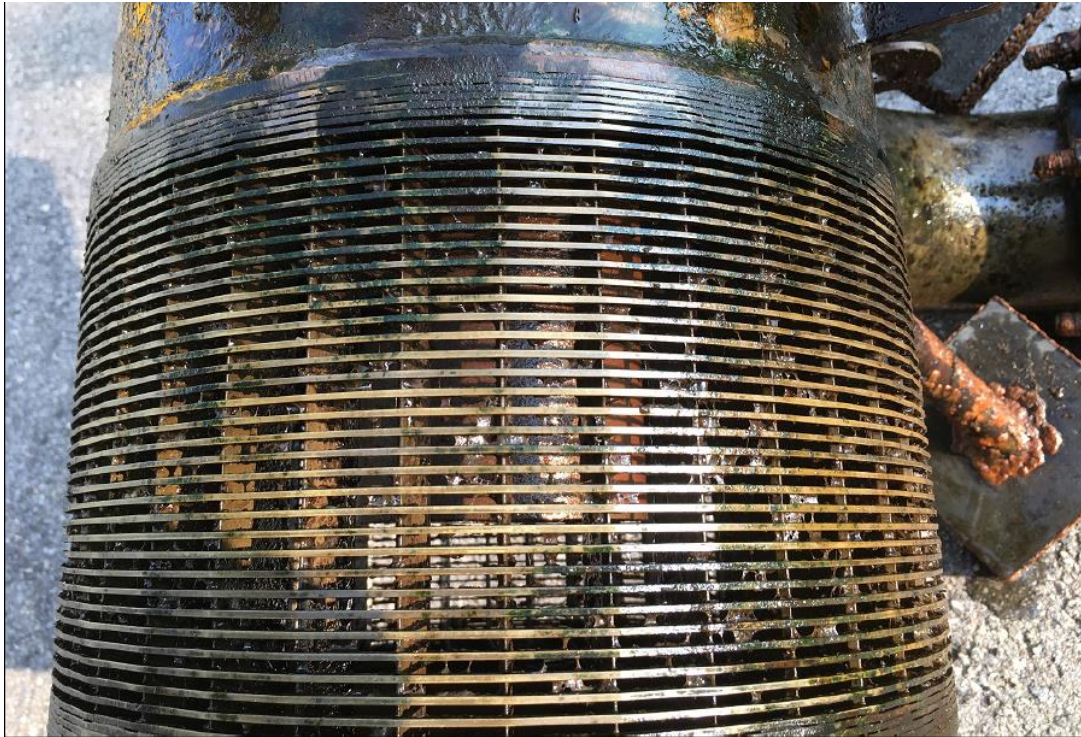
Figure 7 – Post-Test Photo of Upstream Portion of Pilot Test Screen
