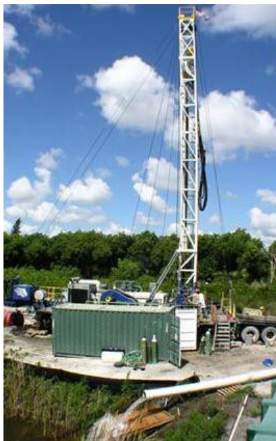
Figure 3-2: Vertical well during construction
