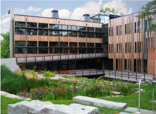
Figure 2 View of new building extension (Photo: Courtesy of Andropogon Associates)
