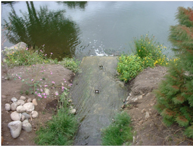
Figure 1 Introduction of reclaimed water to Bell Creek (Photo credit: Gray & Osborne, Inc.)
