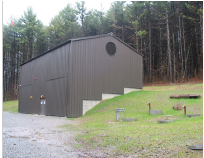
Figure 2 Treatment facility (Photo credit: WEFTEC 2002)
