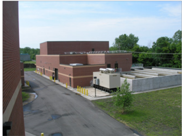
Figure 5-21 Mankato Water Reclamation Facility
