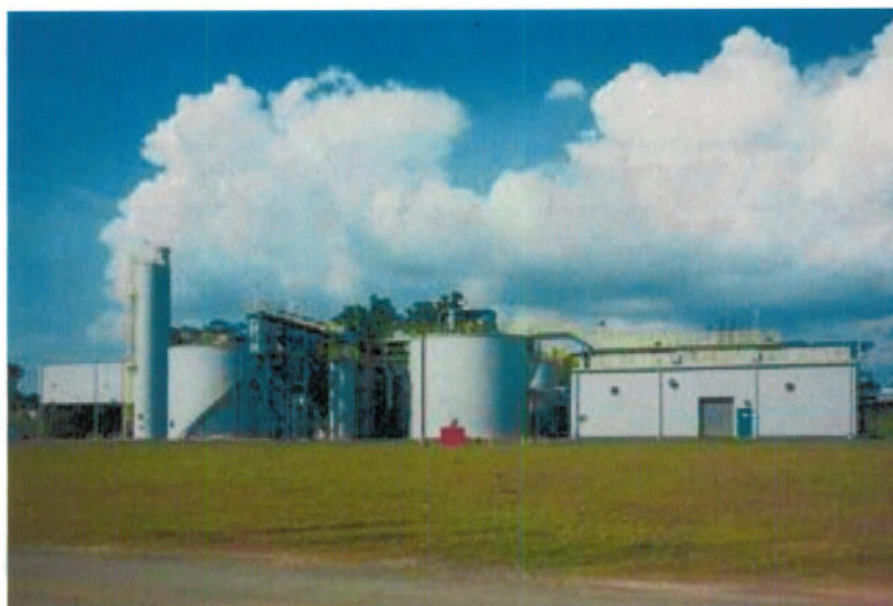
The new bioreactor wastewater treatment system at Allen Station.
