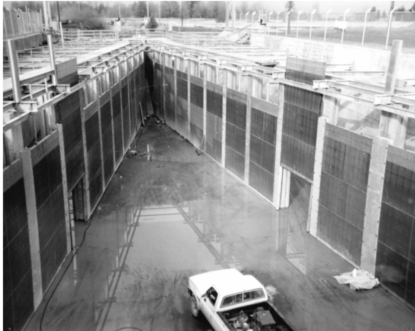
Figure 10-7 White River angled screen diversion system (courtesy of U.S. Filter — Johnson Screen)
