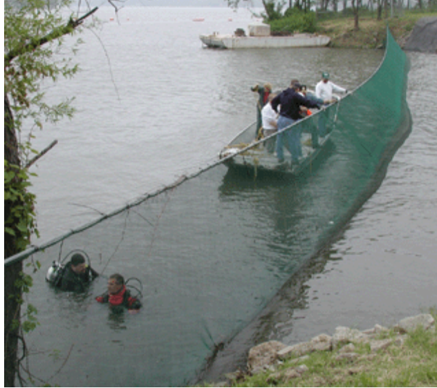
Figure 6-1 Dallman barrier net installation 2003
