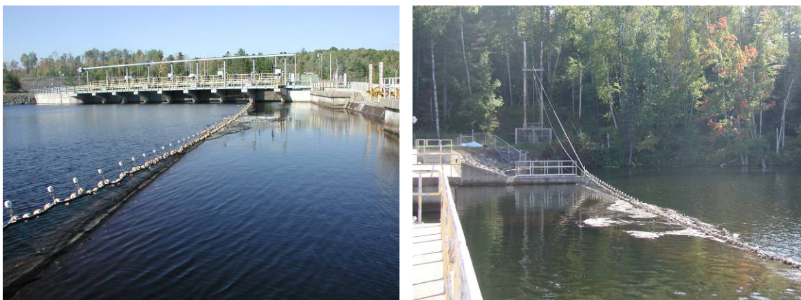
Figure 6-8 Brule barrier net
