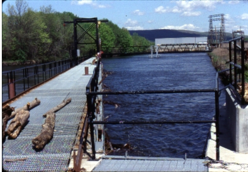
Figure 12-7 Holyoke louver system (photo courtesy of Alden)
