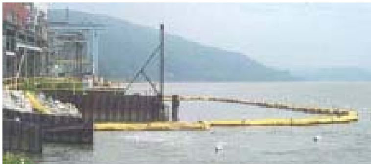
Figure 4.16 Gunderboom® MLEST™ Deployed at Lovett Generating Station
