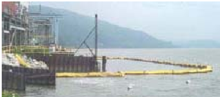
Figure 4.16 Gunderboom® MLES™ Deployed at Lovett Generating Station
