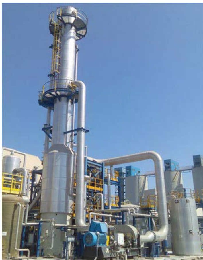
WFGD ZLD System at ENEL Sulcis, Italy, showing Brine Concentrator and Mechanical Vapor Compressor in the foreground. Photo courtesy: Aquatech International.
