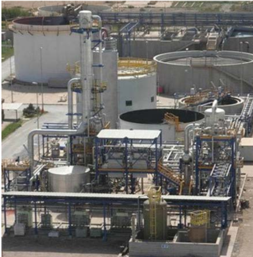
WFGD ZLD System at ENEL Sulcis, Italy. Chemical dosing systems in the foreground, Brine Concentrator the the left, Belt Filter Press at center, Softeners at upper right, and Crystallizer to Center-Right. Courtesy of Aquatech International.
