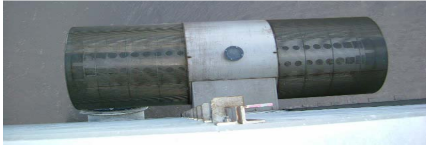
Figure 2-1: Hendrick Wedgewire Intake Screen (Attachment D1)
