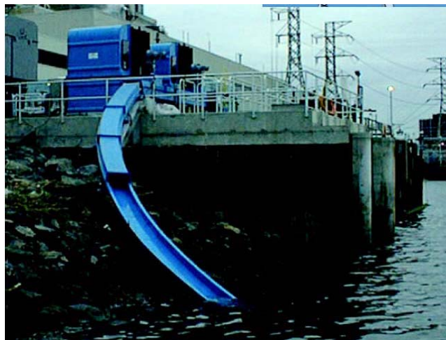
Figure 4-3: Traveling Screens with Fish Sluiceway ( www.glv.com )
