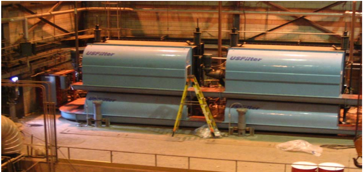
Figure 4-2: Dual Flow Traveling Screen Installation ( www.siemens.com )
