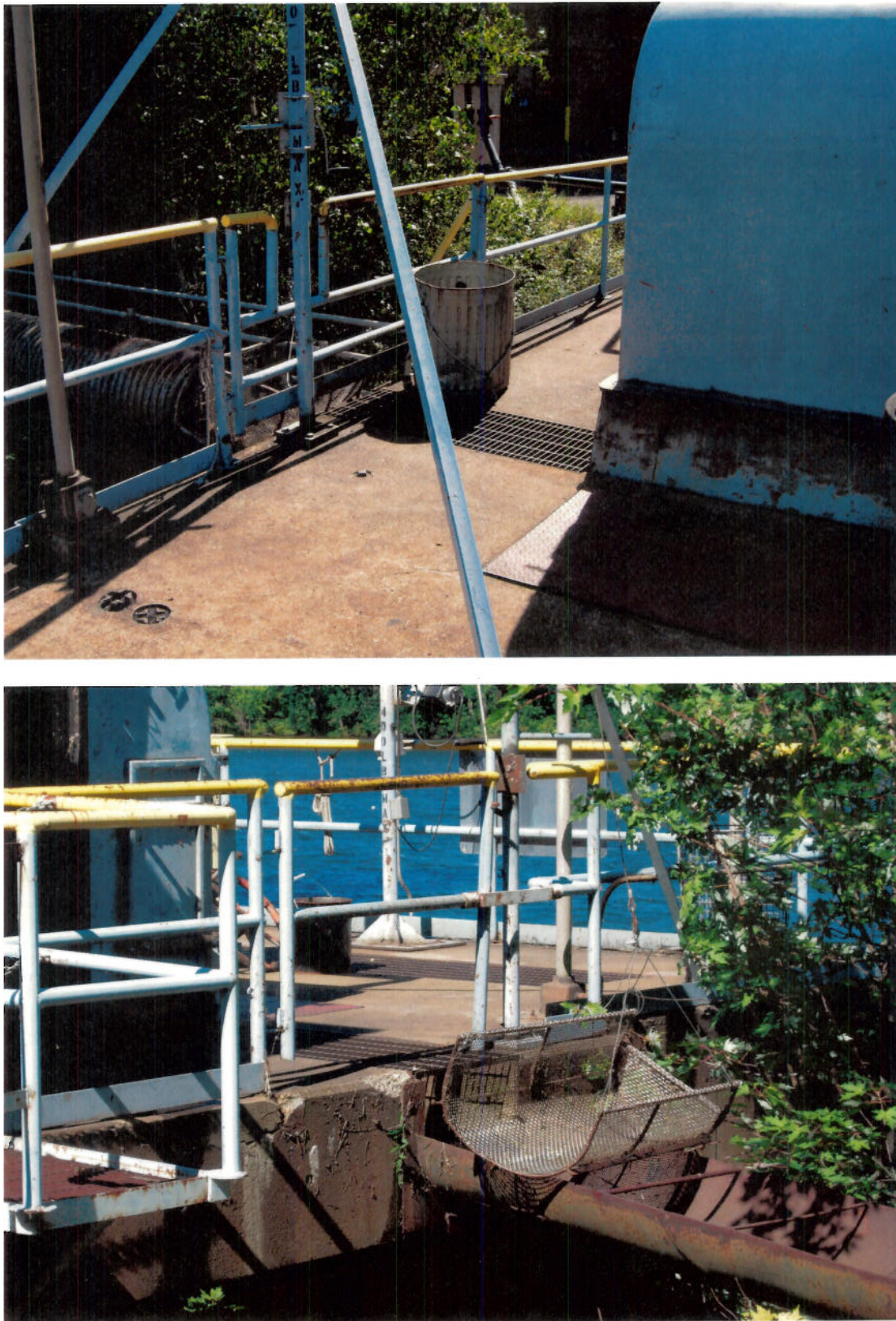
Figure 2-6. Impingement sample baskets at downstream end of debris sluice at Units 1 (top) and 2 (bottom) of Merrimack Station.
