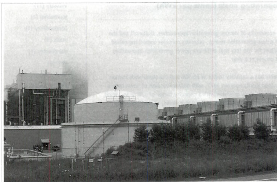
Newington Energy's 606 MW Natural Gas Facility in Newington, NH
