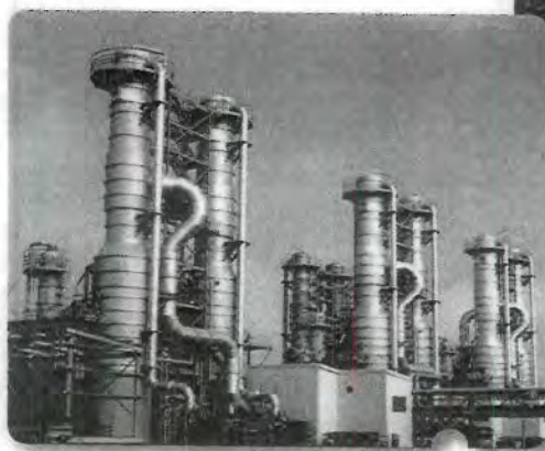
World's Largest Produced Water Evaporator System
