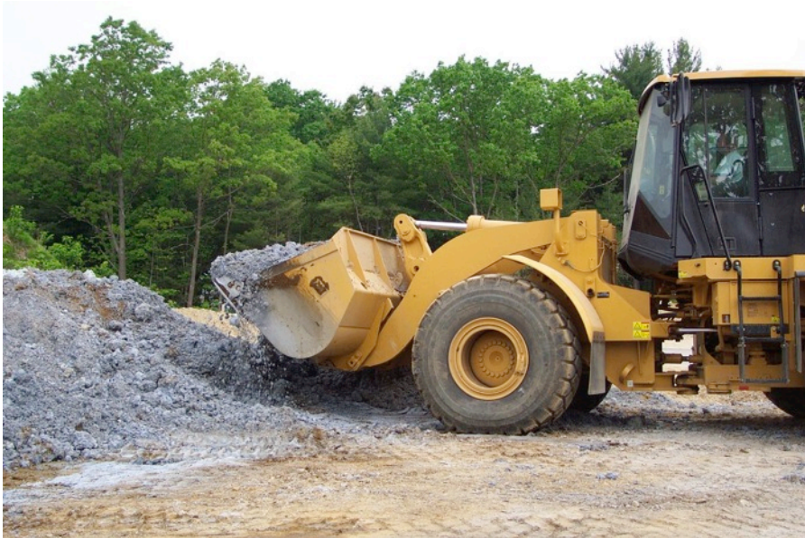
Topsoil blending with paper mill residuals and biosolids, central MA, 2006
