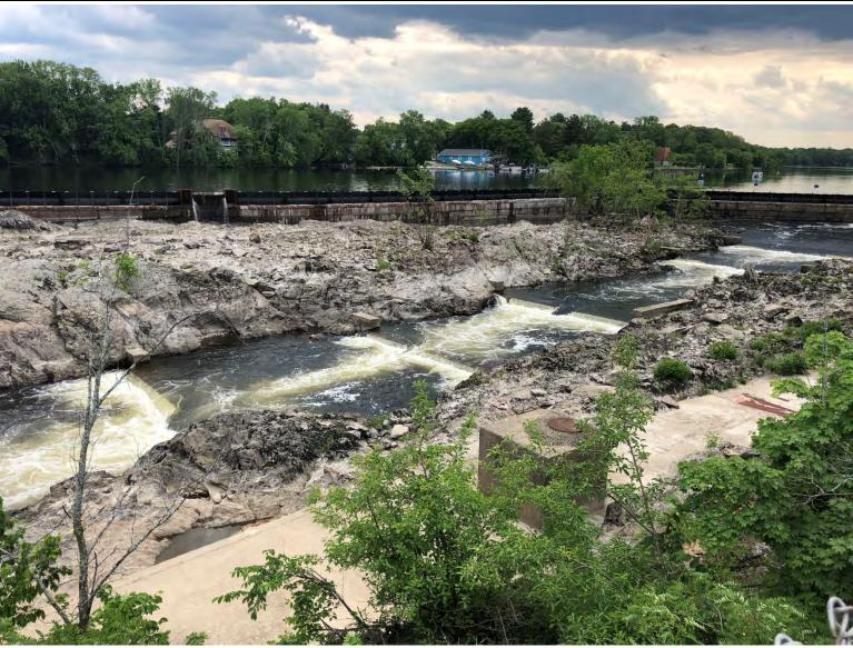
Figure 2–3. Photo of the six concrete flow control weirs located within the Project bypassed reach and downstream of the entrance to the Pawtucket Dam vertical slot fishway.
