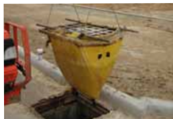
Removed Siltsack® is now ready for cleanout.
