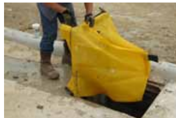
Slide Siltsack® over opposite side of grate.
