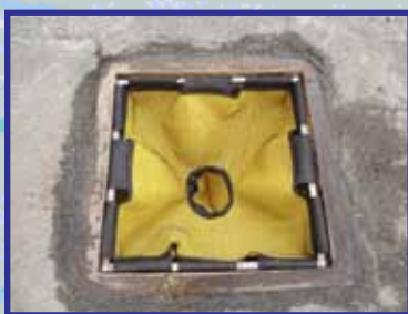
Adjustable frame installed. Adjusts from 16x24 to 24x36.
