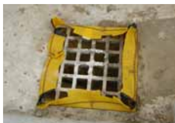
Installed Siltsack®.
