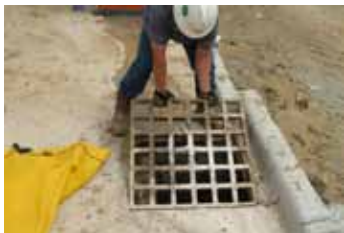
Remove grate from catch basin.
