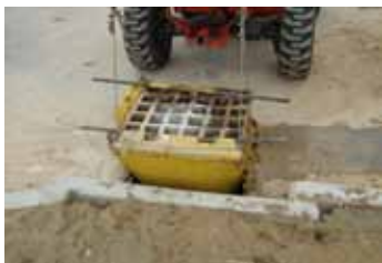
Slowly remove Siltsack® from inlet.
