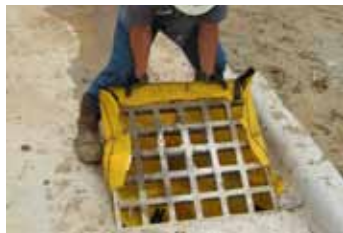
Slide Siltsack® over one side of grate.
