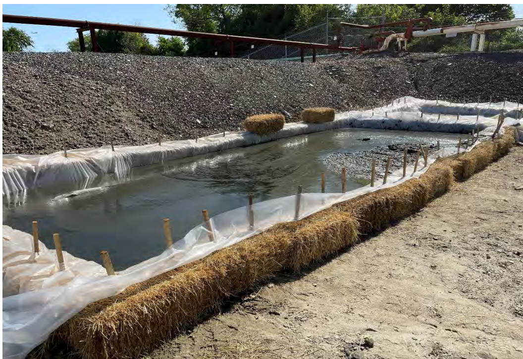
PHOTO 8: View of accumulated removed sediment and storage containment area.
