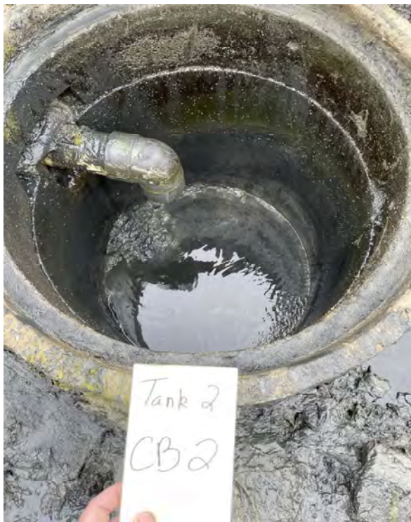
PHOTO 2: Catch Basin (CB-2) following clean out within Tank 2; typical.
