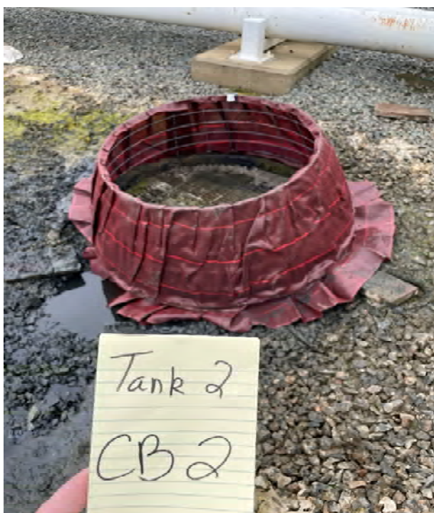
PHOTO 4: CB-2 with grate and sediment control device installed upon completion; typical.
