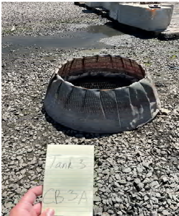
PHOTO 7: CB-3A with grate and sediment control device installed upon completion; typical.
