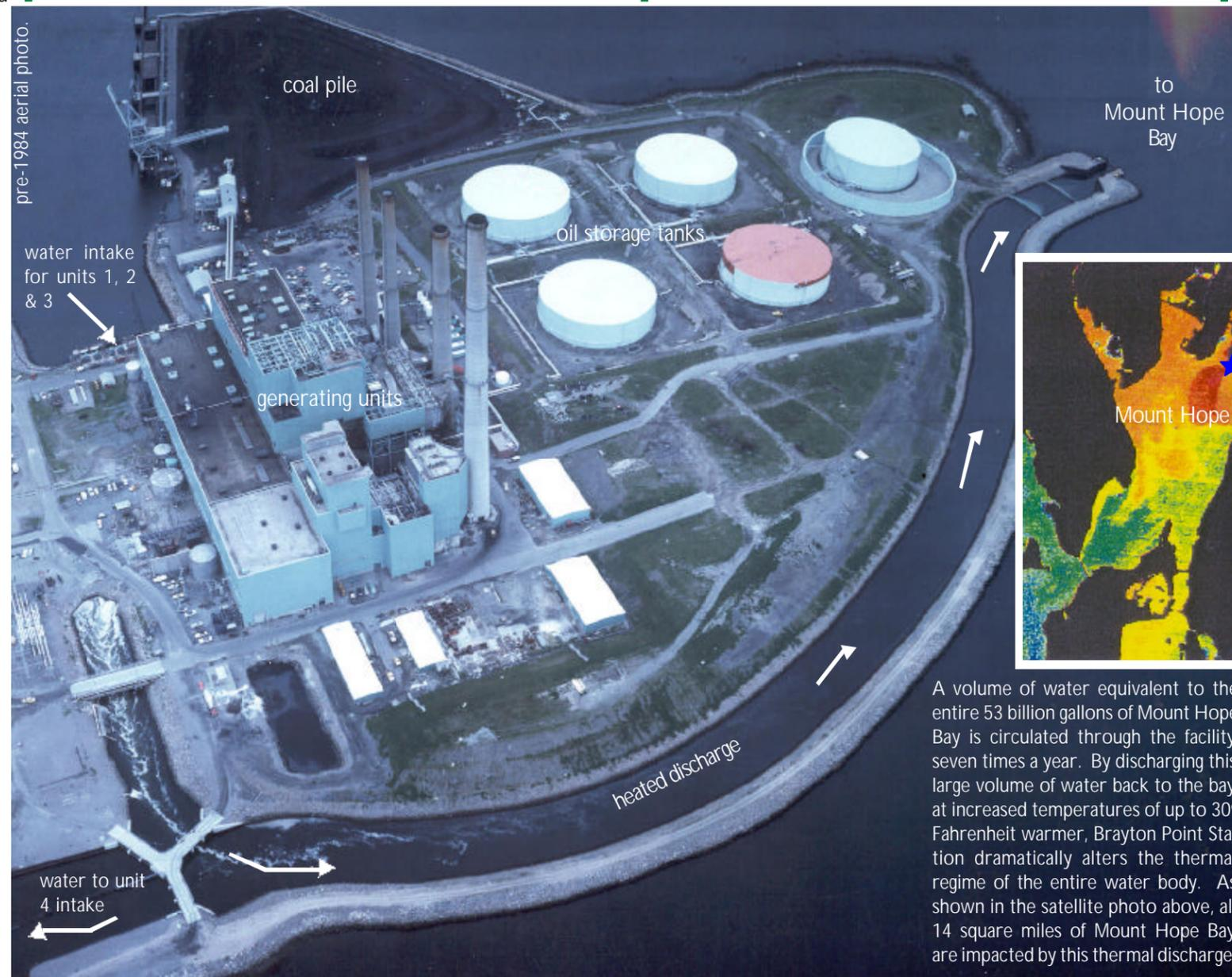
A volume of water equivalent to the entire 53 billion gallons of Mount Hope Bay is circulated through the facility seven times a year. By discharging this large volume of water back to the bay at increased temperatures of up to 30° Fahrenheit warmer, Brayton Point Station dramatically alters the thermal regime of the entire water body. As shown in the satellite photo above, all 14 square miles of Mount Hope Bay are impacted by this thermal discharge.
