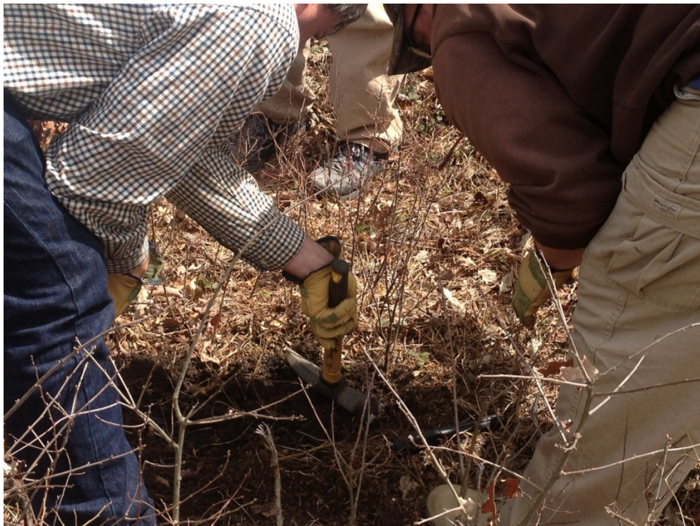
Photo 2 – Clearing surface vegetation and root mass
