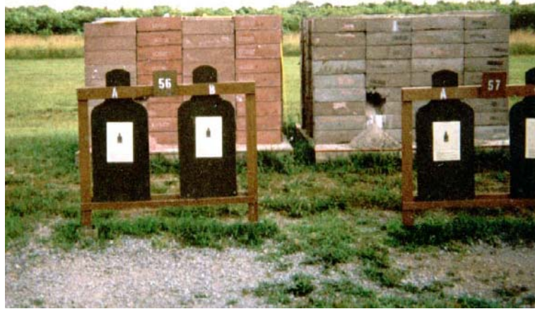
Figure 2-4. Example of Modular SACON® Bullet Containment System (ESTCP 1999)
