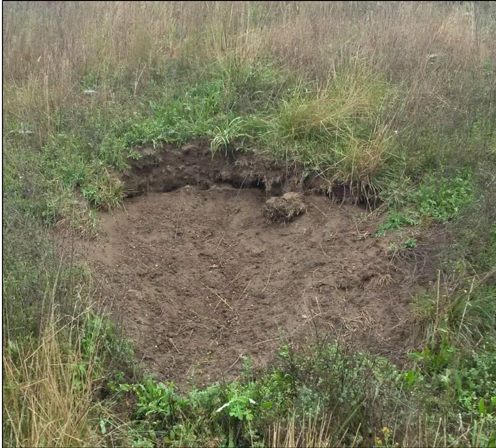
Figure 6. India Range, Top Soil Bullet Pocket, Camp Edwards, Massachusetts (Note: sand visible, needs maintenance to reduce erosion for berm integrity)
