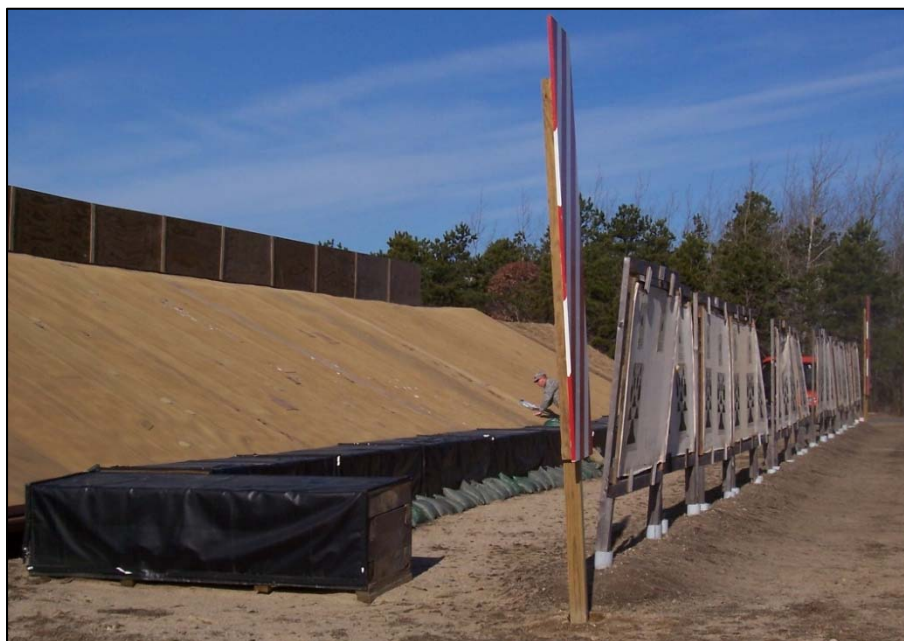
Figure 13. Tango Range Top Cover Inspection, Range Control Camp Edwards, Massachusetts.
