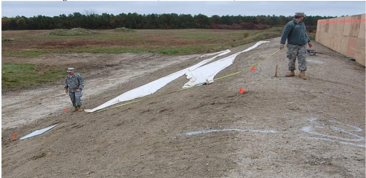
Figure 13. 100 Meter GTL (300m Earthen Berm) on 25 October 2010
