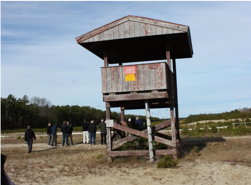
Figure 1: Existing control tower structure
