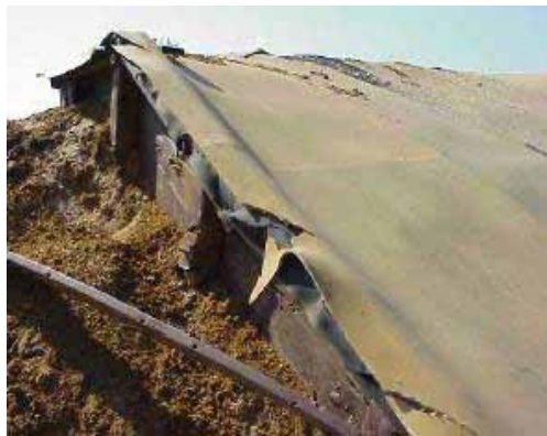
Figure 4-5. Example of Damage to STAPP™ Support Frame (photo not taken at Camp Edwards)
