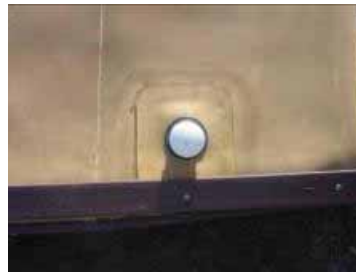
Figure 4-6. Port Access for Water Inspection and Removal
