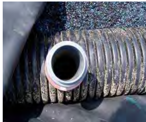
Figure 3-4b Perforated Pipe & Rubber Granules
