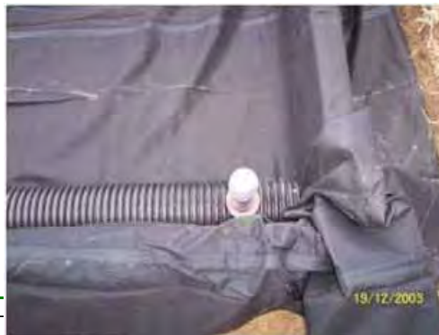
Figure 4-4. Internal Water Reservoir System
