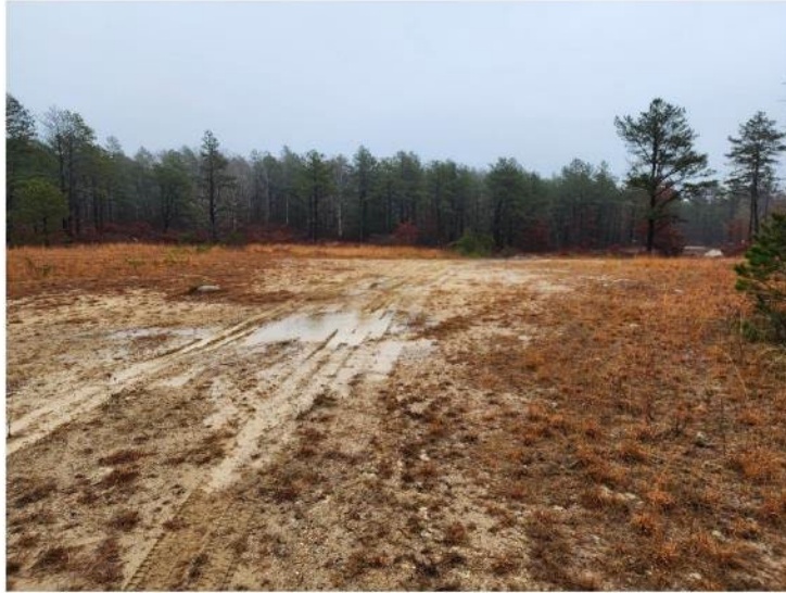
Figure 5: Rutting and puddling at BP20 (picture location 1).
