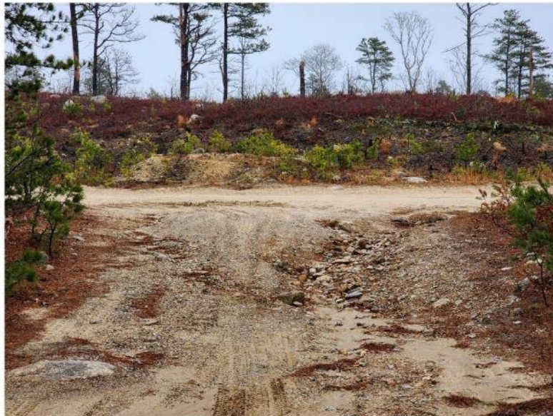
Figure 2: Erosion and rutting occurring on entry road 2 for BP24.
