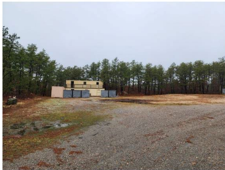
Figure 4: Puddles formed at SVL6.
