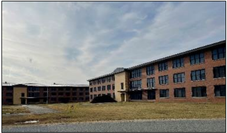
Photograph 5-1 Two of Camp Edwards's barracks with new, metal roofs.
