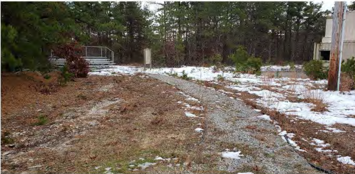
Figure 2: Erosion control at SVL 3, no major erosion since 2017.
