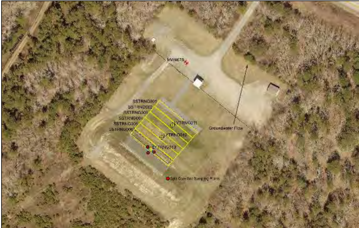
Tango Range with STAPP bullet catcher system, Camp Edwards, Massachusetts LY=Lysimeter, MW=Monitoring Well, SS=Soil Sample
