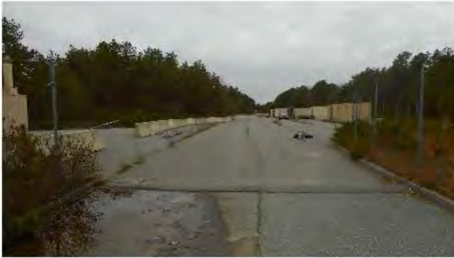
Figure 1: Fence replacement in progress at SVT. 3.
