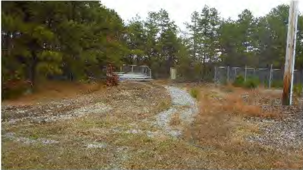
Figure 3: Erosion control at SVI. 3, no additional erosion since 2017.
