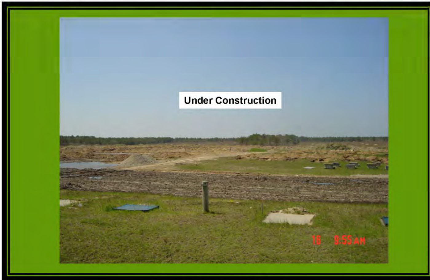
Overview Photo: S Complex
