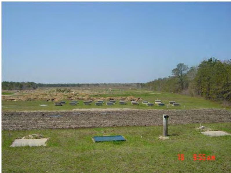
Figure 5-10. S Complex Modernization
