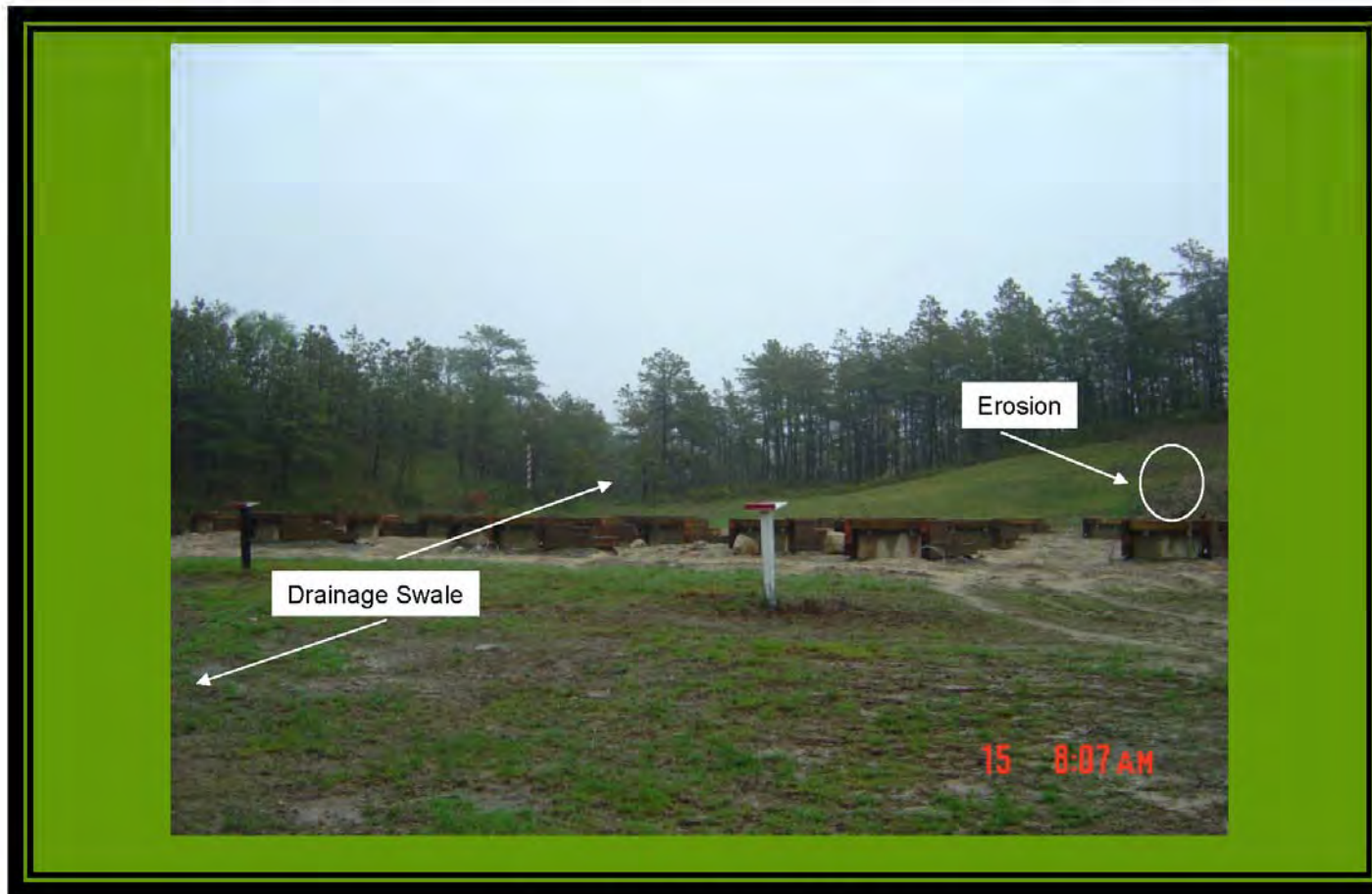
Overview Photo: E Range
