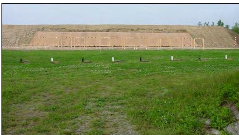
Figure ES-6. Bullet Containment System at T Range
