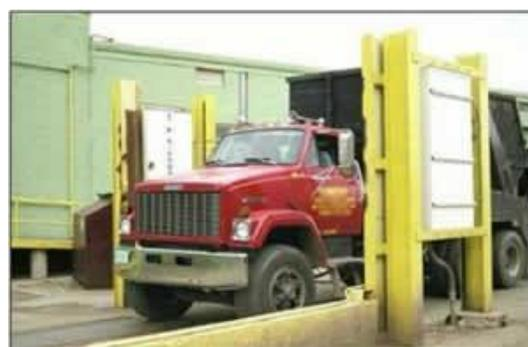
Portal monitors detect radiation in batches of scrap metal.
