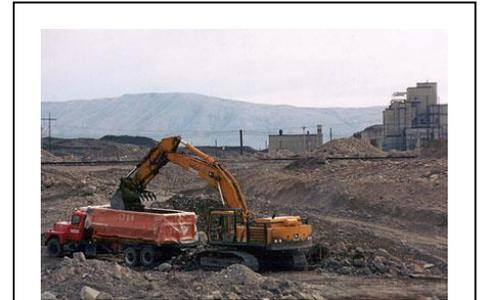
Contaminated soil being loaded into a truck with a former plutonium production reactor in the background.
