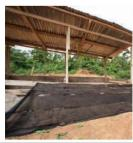
9. Keep fabric tight both vertically and 10. Continue attaching around perimeter of Special Conditions shelter. Measure, cut and attach a separate piece of fabric to the gate. Cut fabric if necessary around other construction features.
