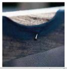
5. Hammer 1 in (3 cm) nails through fabric leaving about ½ in (1.5 cm) of nail protruding from board. Bend nail over, securing the fabric
