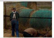
Keep fabric tight both vertically and 10. horizontally. Do not let fabric sag. Do not stretch. Make sure there are no gaps where sections join.
