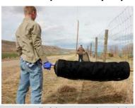
Unroll fabric. Cut desired length (plus additional 1 ½ ft. (50 cm)), then roll the cut piece so it will be easier to handle during installation. Shake loose dirt from fabric before installing.
