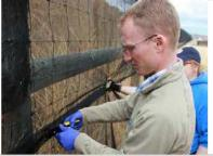
Once top is secure for a few yards (meters) pull fabric tight from below and fasten at bottom. Attach one section top and bottom then unroll as needed.
