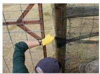
Start attaching at edge of entry gate of shelter by securely fastening from bottom to top by nailing for wooden structures and using zip ties, plastic clips or hog rings for wire or metal structures.
