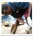
8. Once top is secure for a few yards (meters) pull fabric tight from below and hammer nails at bottom. Attach one section top and bottom then unroll as needed.
