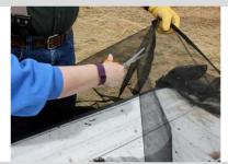
Continue attaching perimeter of shelter. Measure, cut and attach a separate piece of fabric to the gate. Cut fabric if necessary around other construction features.
