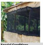
Install fabric flush to top of concrete or brick wall. Ensure that no space is left open.
