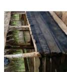
Keep fabric tight both vertically and horizontally. Do not let fabric sag. Do not stretch. Make sure there are no gaps where sections join.
