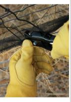
ю. Attach fastener through fabric and structure, securing the fabric. ы.
