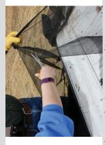
perimeter of shelter. Measure, cut and attach a separate piece of fabric to the gate. Cut fabric if necessary around other construction around attaching Continue features. 10.
