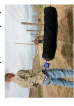
(plus additional 1 % ft. (50 cm)), then roll the cut piece so it will be easier to handle during Unroll fabric. Cut desired length installation. Shake loose dirt from fabric before installing. ч.
