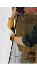
Continue fastening on top. Space 2 -2 ½ ft. (60 -70 cm) apart. Keep fabric tight. ~ Roll out fabric as needed. Make sure it is straight and tight against structure of shelter.
