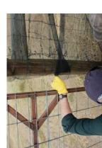
Start attaching at edge of entry gate of shelter by securely fastening from bottom to top by nailing for wooden structures and using zip ties, plastic clips or hog rings for wire or metal structures. ÷.
