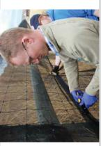
Once top is secure for a few yards pull fabric tight from below and fasten at bottom. Attach one section top and bottom then unroll as needed. (meters) ŵ
