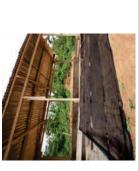
Continue attaching around perimeter of shelter. Measure, cut and attach a separate piece of fabric to the gate. Cut fabric if necessary around other construction features.
