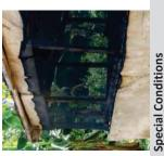
Install fabric flush to top of concrete or brick wall. Ensure that no space is left open.
