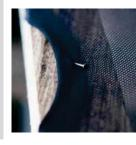
Hammer 1 in (3 cm) nails through fabric leaving about % in (1.5 cm) of nail protruding from board. Bend nail over, securing the fabric
