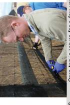
Once top is secure for a few yards pull fabric tight from below and fasten at bottom. Attach one section top and bottom then unroll as needed. (meters) ∞
