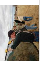
Roll out fabric as needed. Make sure it is straight and tight against structure of shelter. 9
