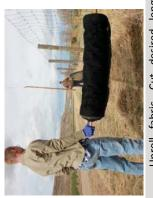
(plus additional 1 % ft. (50 cm)), then roll the cut piece so it will be easier to handle during installation. Shake loose dirt from fabric Unroll fabric. Cut desired length before installing.
