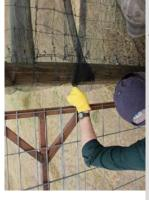
Start attaching at edge of entry gate of shelter by securely fastening from bottom to top by nailing for wooden structures and using zip ties, plastic clips or hog rings for wire or metal structures.
