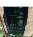
Install fabric flush to top of concrete or brick wall. Ensure that no space is left open.
