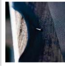
Hammer 1 in (3 cm) nails through fabric leaving about ½ in (1.5 cm) of nail protruding from board. Bend nail over, securing the fabric
