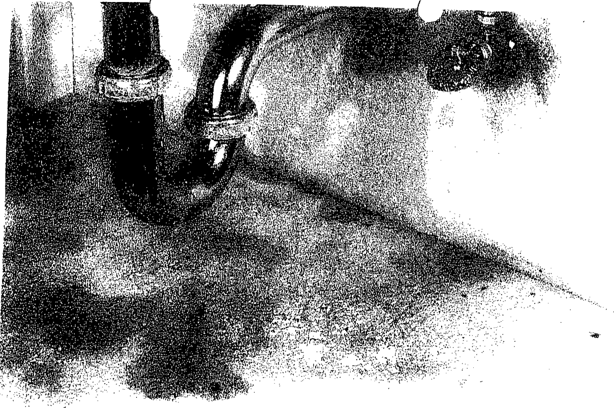
sink before Image_0077.jpg
