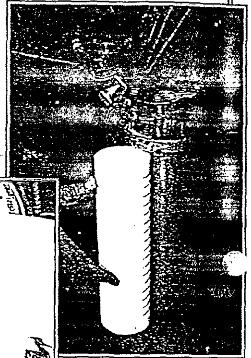
Regularly replace in-line filters.
